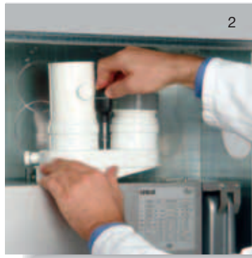
Smoke outlet installation
