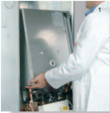
Boiler positioning into the built-in box
