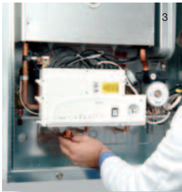
Hydraulic and electric connections
