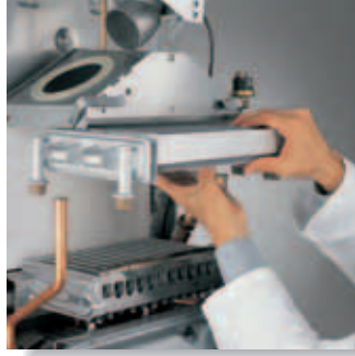
Heat exchanger removal by front ward sliding
