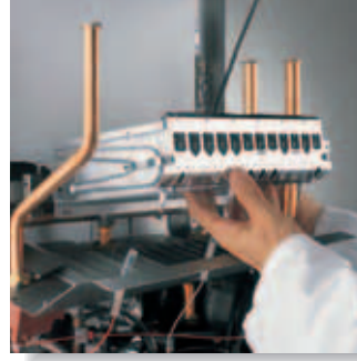
Burner removal by front sliding without remaining the gas train
