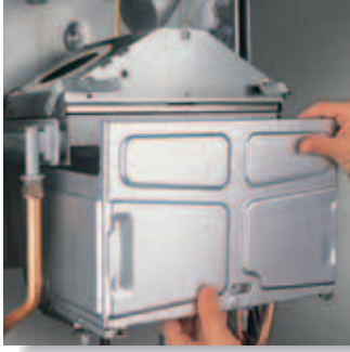
Opening of the combustion chamber with release levers
