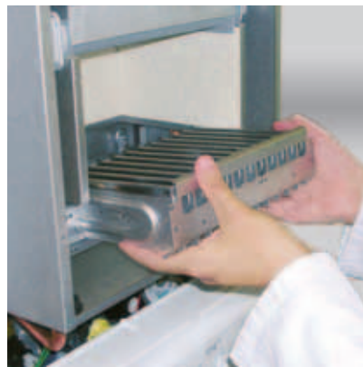
Burner removal by front sliding without removing the gas train
