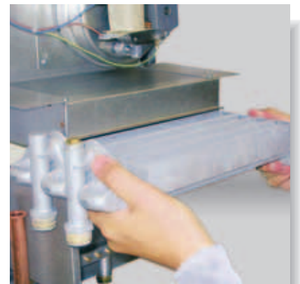
Heat exchanger removal by front ward sliding
