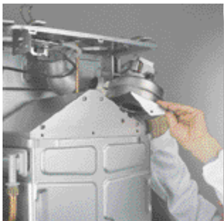
Fan frontward removal with removal of just one screw
