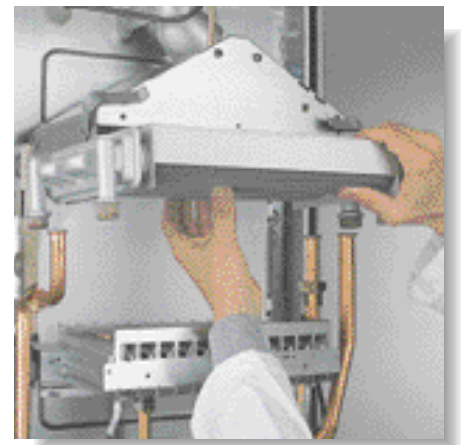
Heat exchanger removal by front ward sliding
