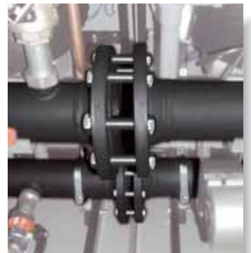
Simple installation (detailed view flange/flange)
